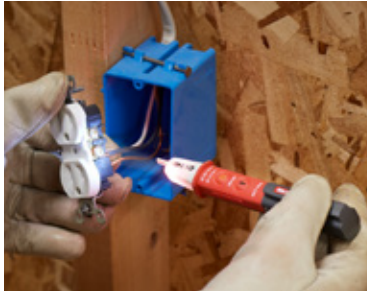
Test wires for AC voltage
