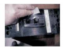
Clean oils and other debris from the circuit breaker panel face using the provided Alcohol wipes
