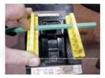
Align the yellow mounting rails on each side of the breaker switch with the marks made in step 2. Peel the backing from the "High Bond" permanent tape and lace the rails onto the cleaned surface.
