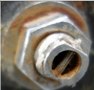
COMPONENTS AND LEAKS
